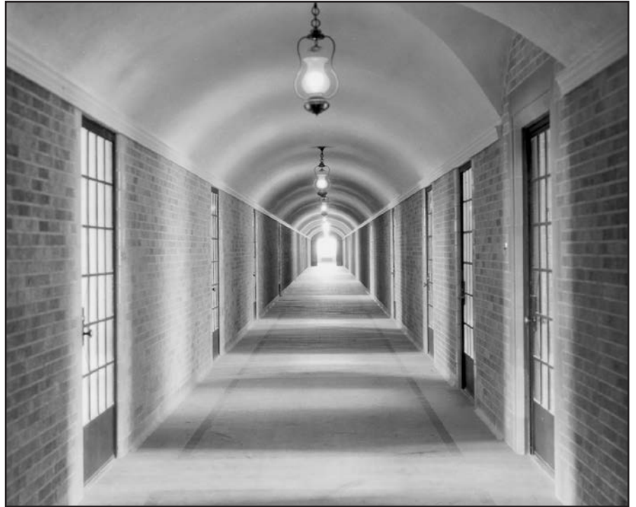
Corridor, showing laboratory doors of steel with glass panels
